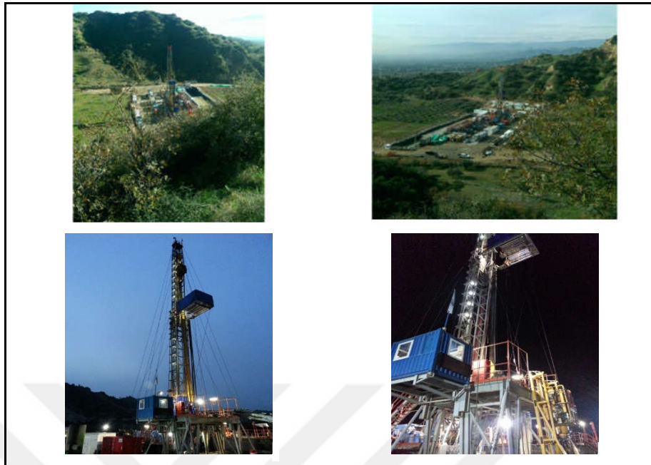
Figure 3.16. Views of the KS-2 location and drill rig.
