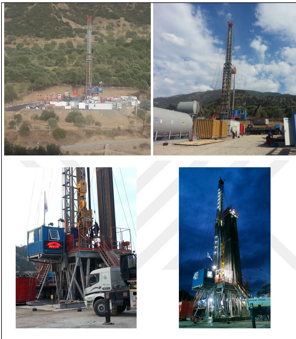
Figure 3.12. View from KS-1 borehole location and drill rig
