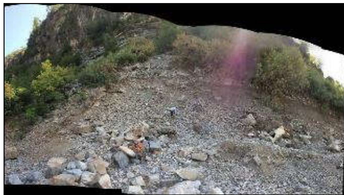
Figure 7.11. Terziler Road, TY2 location, Permian marbles.
