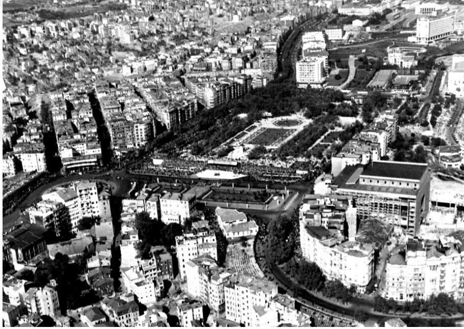
Figure 4.7. Aerial view of Taksim, 1960. Source: Google Arts and Culture, from ( artsandculture.google.com/asset/aerial-view-of-taksim-and-vicinity )
