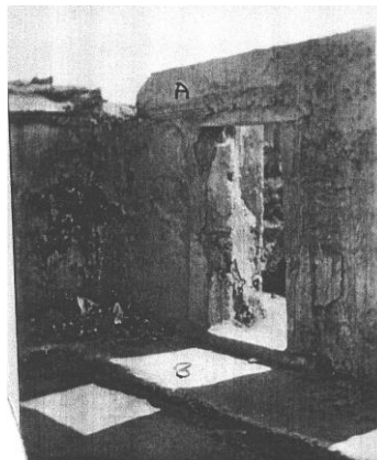
Fig. 248 House C7B 2 , The door between room 2 and room 4, the plaster cornice above the door (A) and bench on the floor (B). (Baird, 2006: fig. 78)
