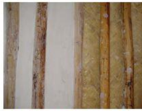
Figure 49 Reconstructed ceiling at Dura (using ancient methods) showing reed matting laid over wooden beams (left side has been plastered).
