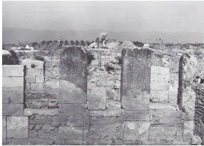
Fig. 107 The House of the Deer, East wall of room A with windows opening to courtyard D (Donnay-Rocmans and Donnay, 1984: Plate LI.3)
