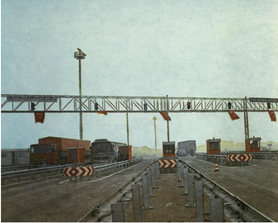
Figure A.12. İzmit – Kirazlı Toll Motorway (source: Bakanlık Bülteni , no. 82 (May, 1984))
