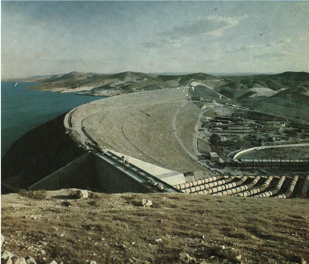
Figure A.1. Atatürk Dam (source: Bakanlık Bülteni , no. 114 (March, 1992))
