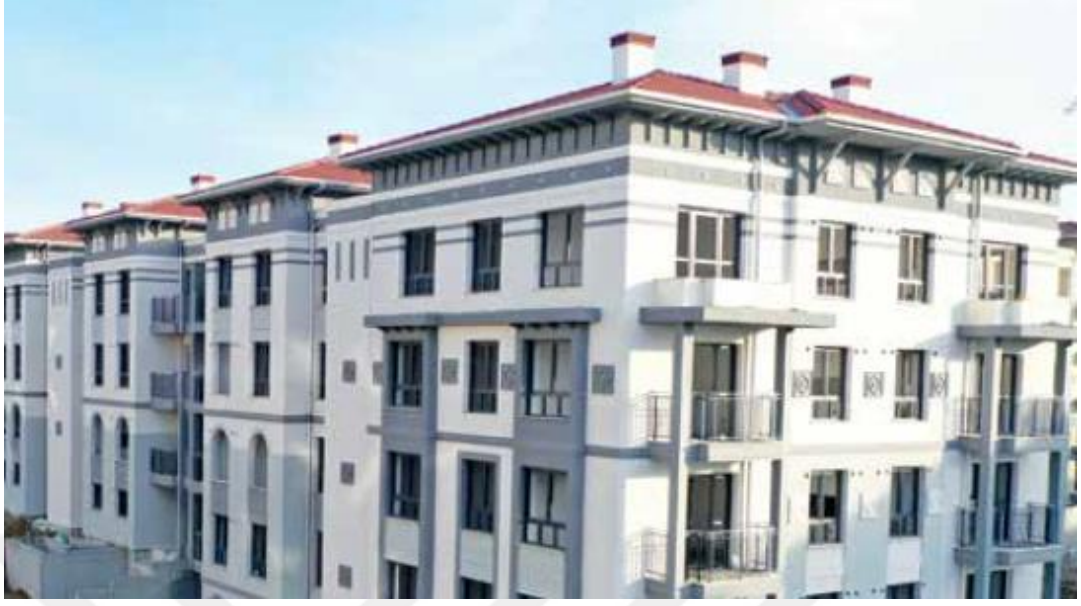
Figure C. 2. İstanbul Esenler Urban Transformation Project (source: Bakanlık Bülteni , no. 145 (March, 2022))
