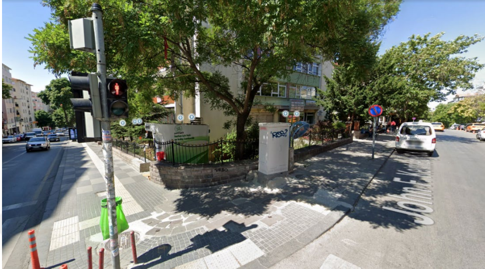
Figure 64. Existing condition of Patch 72 (Google Maps).
