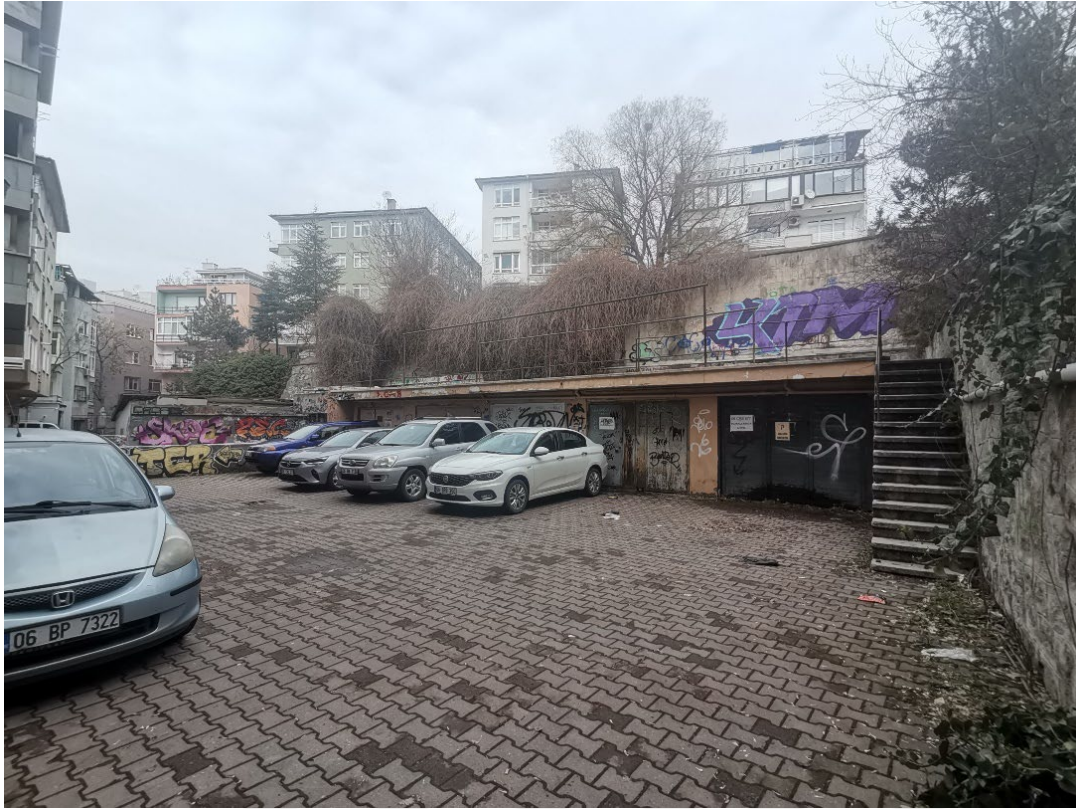
Figure 37. Illegally built closed parking garage.
