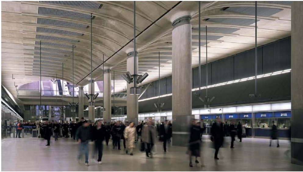
Figure 45 - Canary Wharf Underground Station platform area (Foster+Partners)
