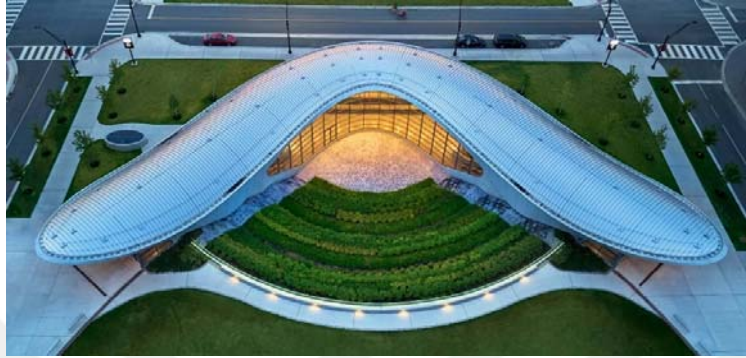
Figure 57 – Top view of York University Station (Foster+Partners)
