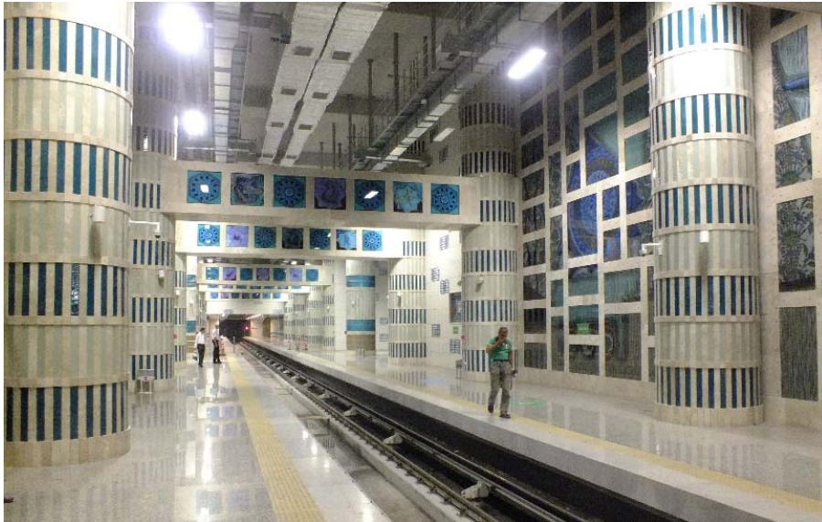
Figure 77 – View of Yenikapı M2 line platform level (Dorsam, 2014b)
