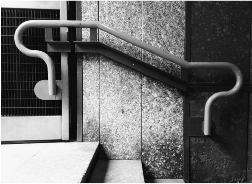
Figure 36 - Milan Subway handrail view with the wall cladding ( Jones, 2016 ).
