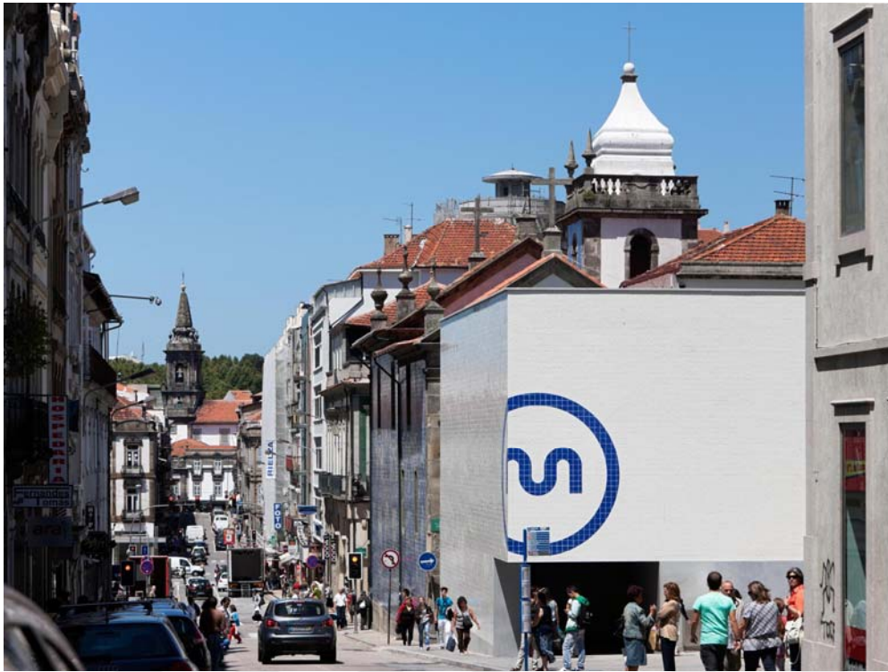
Figure 47 - Bolhao Station entrance building with blue Porto Metro sign (Luis Ferreira Alves)
