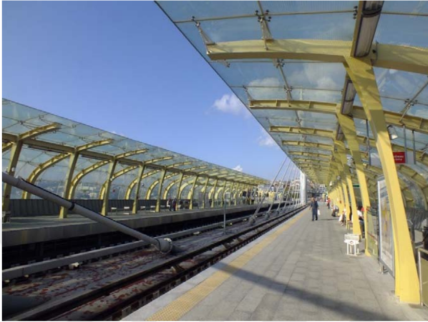
Figure 81 - Haliç Station platform view showing the platform area and the canopy above (Dorsam, 2014a).
