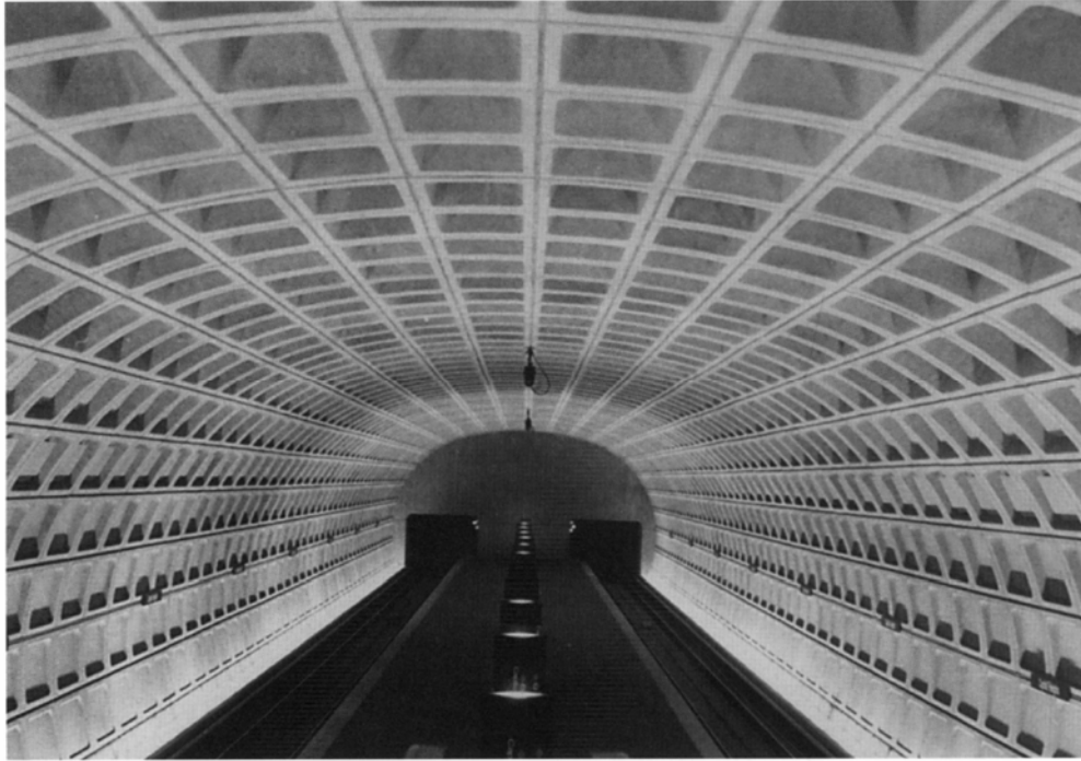
Figure 38 - Washington D.C. subway platform area view ( Miller and Raines, 2000 )
