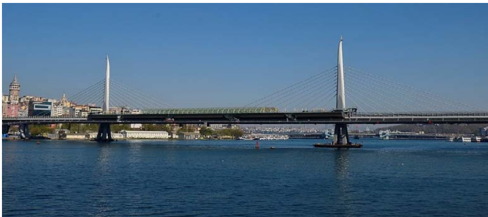
Figure 80 - Haliç Bridge Station at Yenikapı-Hacıosman Line in Istanbul, seen from West (CeeGee, 2014).
