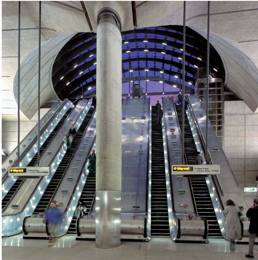
Figure 44 - Iconic glass canopy of Canary Wharf Underground Station in London (Foster+Partners)
