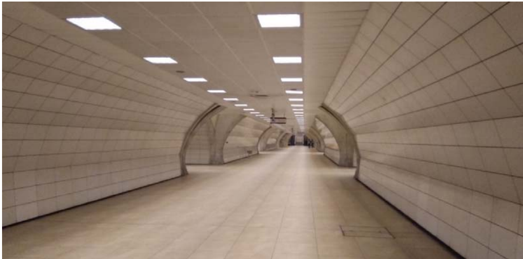
Figure 14 – Central tunnel of Yenisahra Station in Istanbul showing the lack of architectural features (author)
