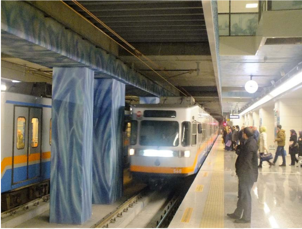
Figure 78 – View of Yenikapı M1 line platform level (Dorsam, 2019)
