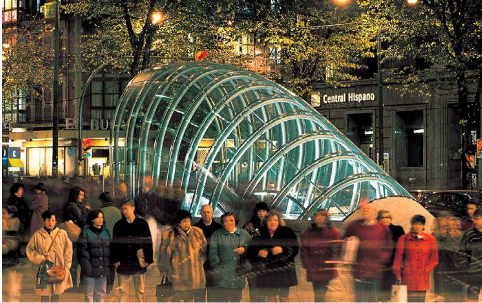
Figure 41 - Glass canopy of Bilbao subway stations (Foster+Partners)
