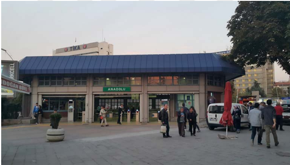
Figure 99 – Anadolu (Tandoğan) station passenger entrance (BurakOtto, 2016b).
