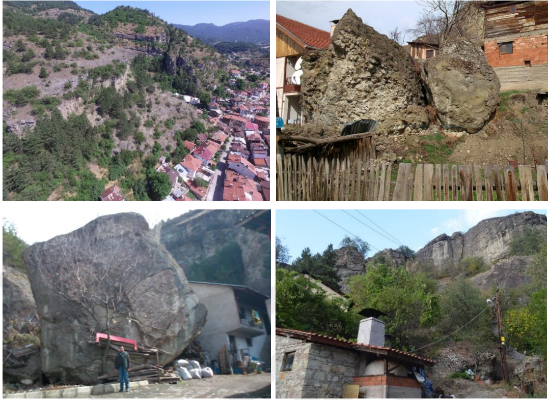
Figure 4: Views from the rock mass of the east side of the Mudurnu valley which shows those houses that are under the threat of the large blocks
