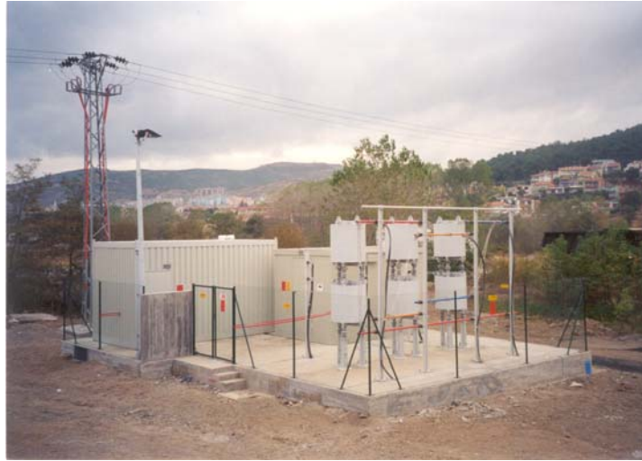
Figure 1.3 SVC-Thyristor Controlled Reactor
