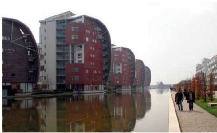
Figure 2.19. A depthless pool in Hertogenbosch acts like a solar panel for the surrounding buildings (Aparicio 2008) [Graaf 2012]
