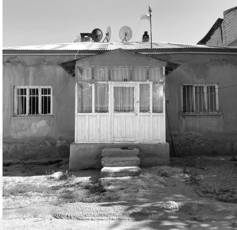
Figure 5-3 An old mudbrick house in Hafziye. Photograph by the author, captured in May 2022.
