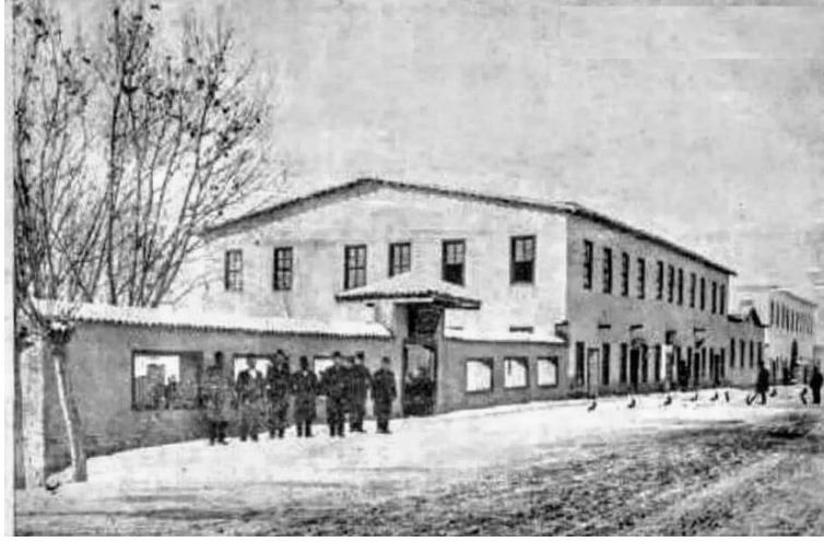
Figure 4-30 An official building in the inner city. 464
