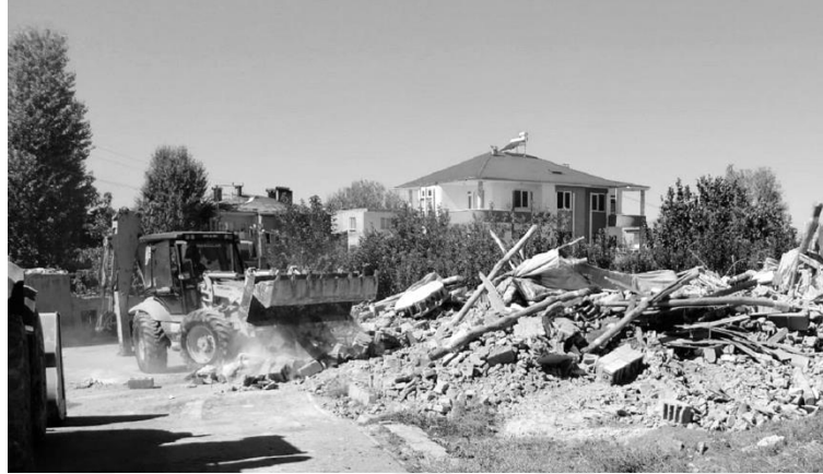
Figure 5-9 Demolition of a shock house in Hacibekir. From a daily newspaper issued on 26 September 2021.
