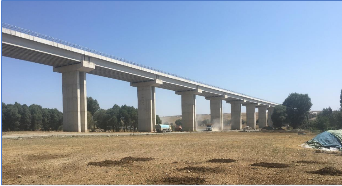
Figure 8: Ongoing Construction of the Ankara-Sivas High-Speed Train Line, Çiğdemli, 08/30/2019
