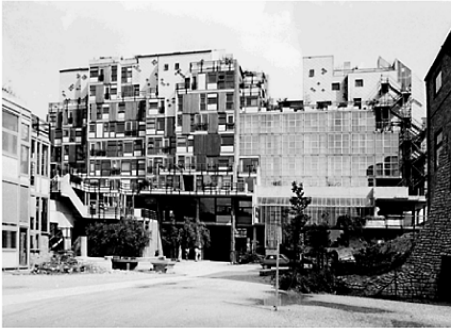
Figure 2-12. A general view of Maison Médicale 110
