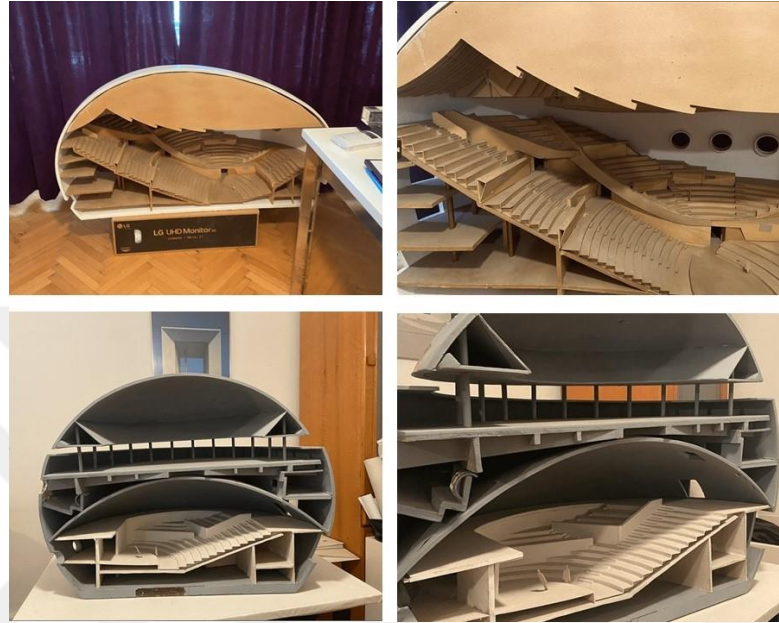
Figure 4.22- Section Model of the Main Concert Hall and Chamber Music Concert Hall made in 1:50 scale, photography by the author.
