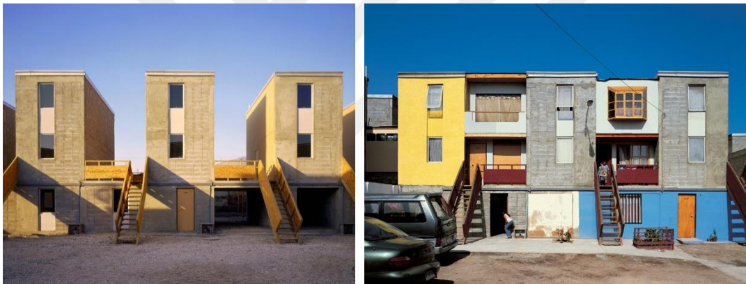
Figure 3.37. Incomplete forms before and after filled in (Accessed August 22, 2022 from https://www.archdaily.com/10775/quinta-monroy-elemental )
