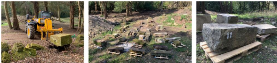
Figure 2.15 Reclaiming, collecting, and numbering stone blocks (Wilton et al., 2025)
