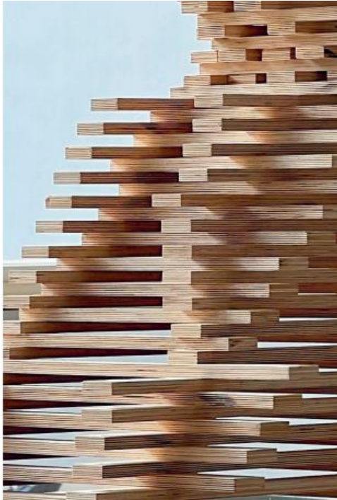
Figure 2.3 Compression-based structure with wooden pieces (Hunkar & Lee, 2023)
