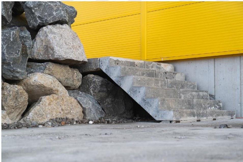
Figure 2.13 Reclaimed stair (Jhons, 2023)
