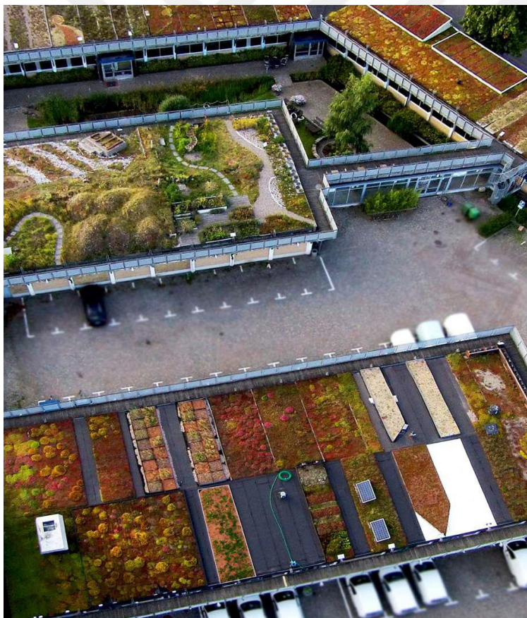
Figure 4.10. Green Roofs in EcoCity Augustenborg (Persson & Mansson, 2021).
