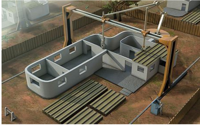
Figure 2.3. Contour Crafting Method (Khoshnevis, 2010)
