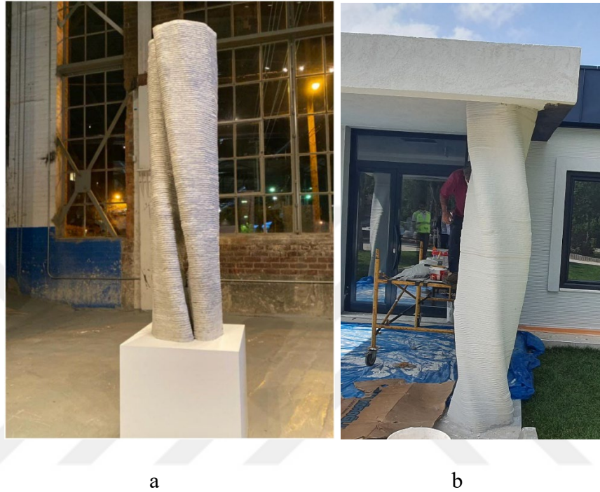
Figure 2.8. (a) Twisted column, University of Michigan (Li et al., 2020), (b) Twisted column, ISTON 3DCP office building entrance.
