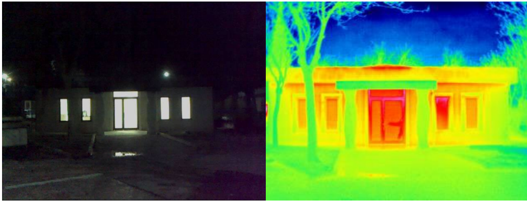
Figure 5.1. The thermal imaging completed between 2-5 am to minimize the convective heat loss
