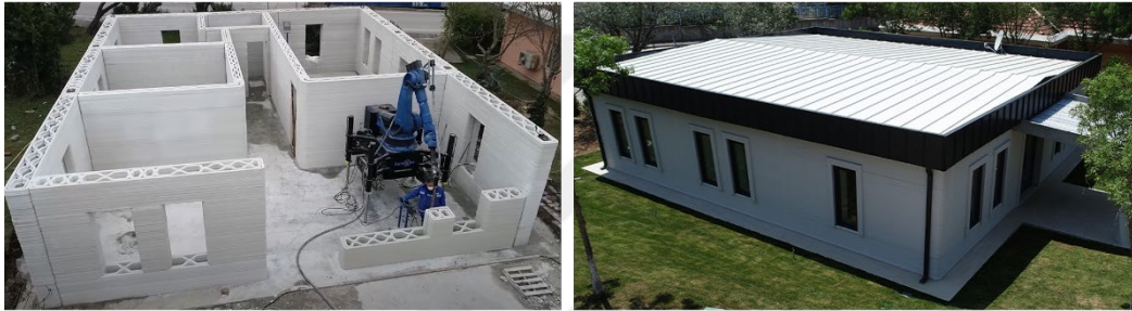
Figure 4.2. Aerial photographs of the 3DCP case building's construction and final phases
