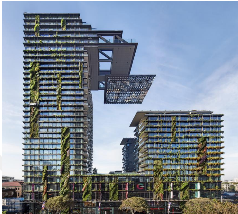
Figure 2.11. One Central Park (Ateliers Jean Nouvel, 2014)
