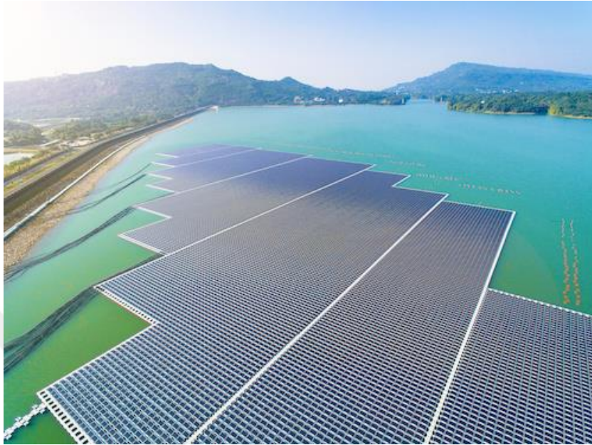
Figure 2.4. Floating PV by Intersolar (intersolar EUROPE, 2023)
