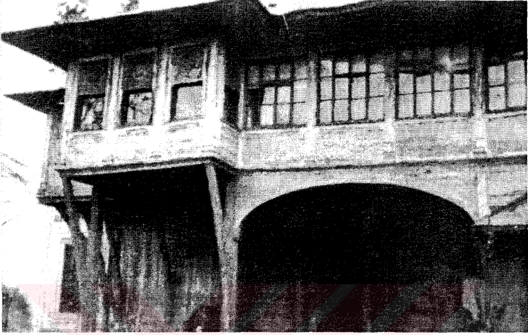
Figure 5.11: Imperial Pavilion of Sultan Mahmud II next to the Beyazıt Mosque
