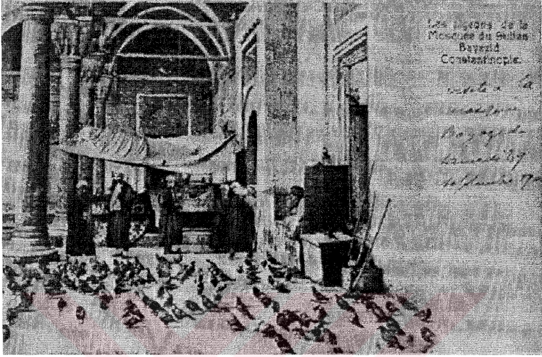
Figure 5.23: Interior Courtyard of Beyazıt Mosque.
