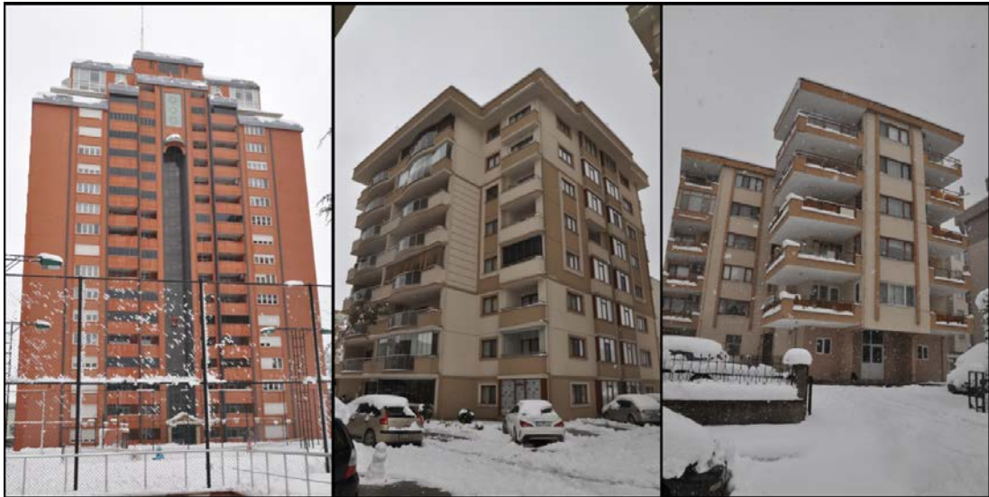
Figure 3.2. Photographs for samples DH, CH and IH system buildings respectively
