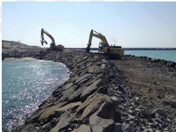
Figure 5.9 Breakwater built by rock
