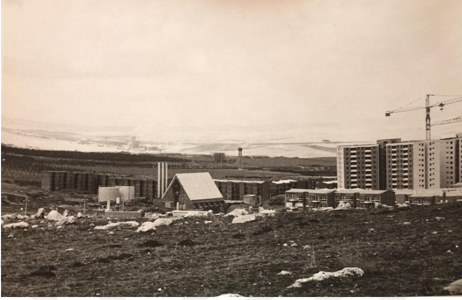
Figure 4.29. A photograph from the construction of five-story and multiple-story İşçi Blokları.
