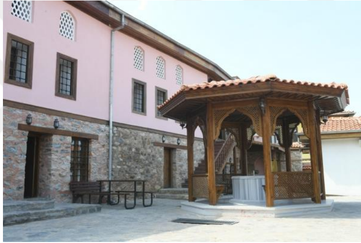
Figure 4.9. Somuncu Baba House, Bakery and Cultural Center
