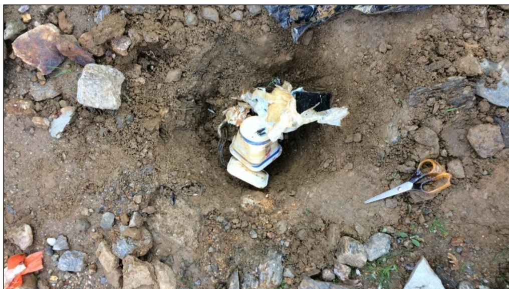
Figure 5.25. Location 3, Benzinlik, water damage.
