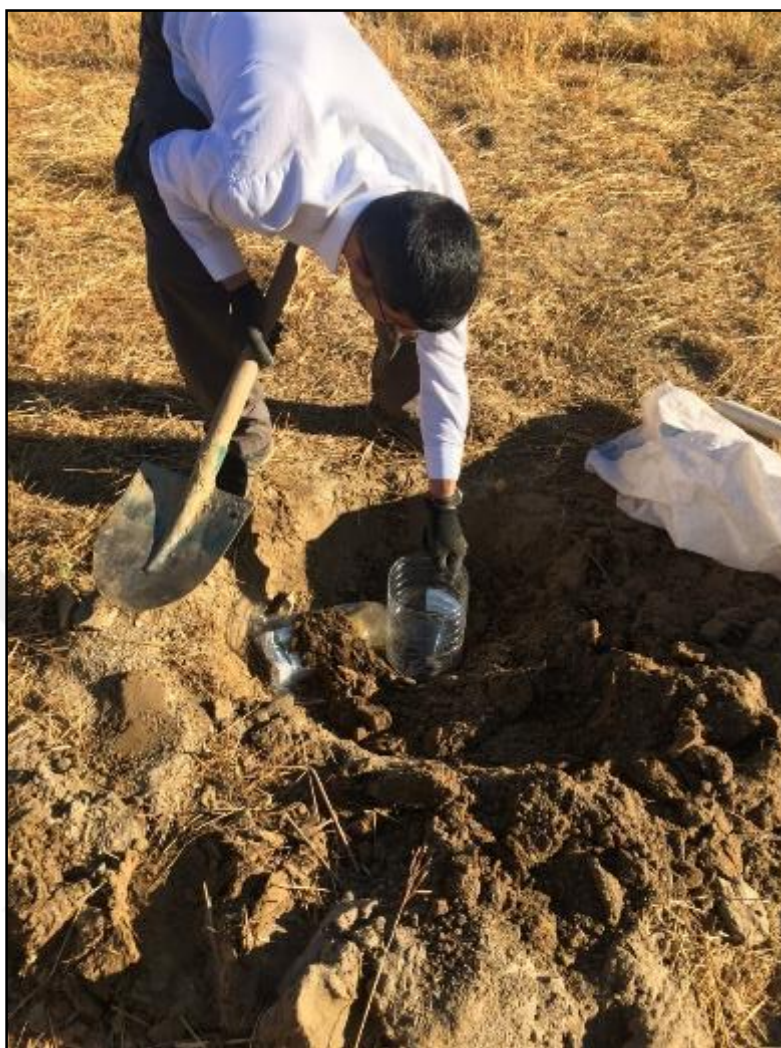
Figure 5.19. Backfilling PVC casing.
