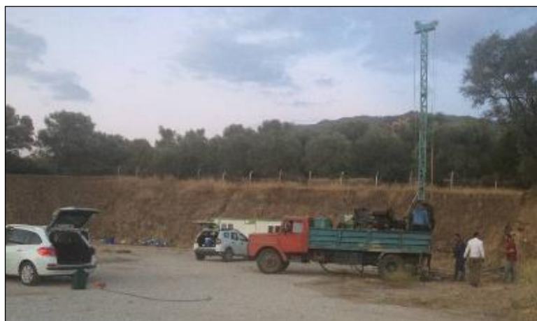
Figure 5.16. KS1 location drilling operation.
